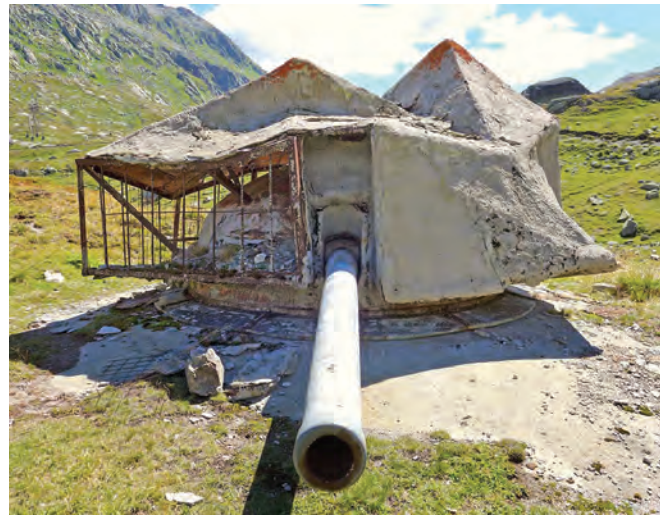
Fort San Carlo: Turret 2, now revealing the construction of its camouflage superstructure
